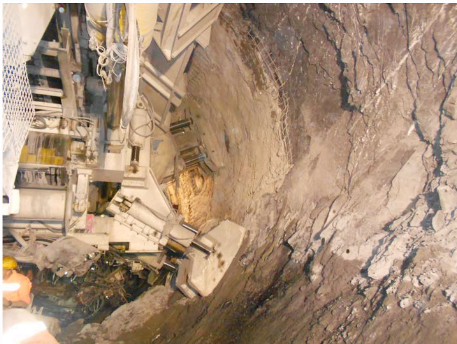
Fig. 2: Example of an open gripper-TBM in Switzerland showing collapsed side-wall within the L1-area providing no protection for the staff.
