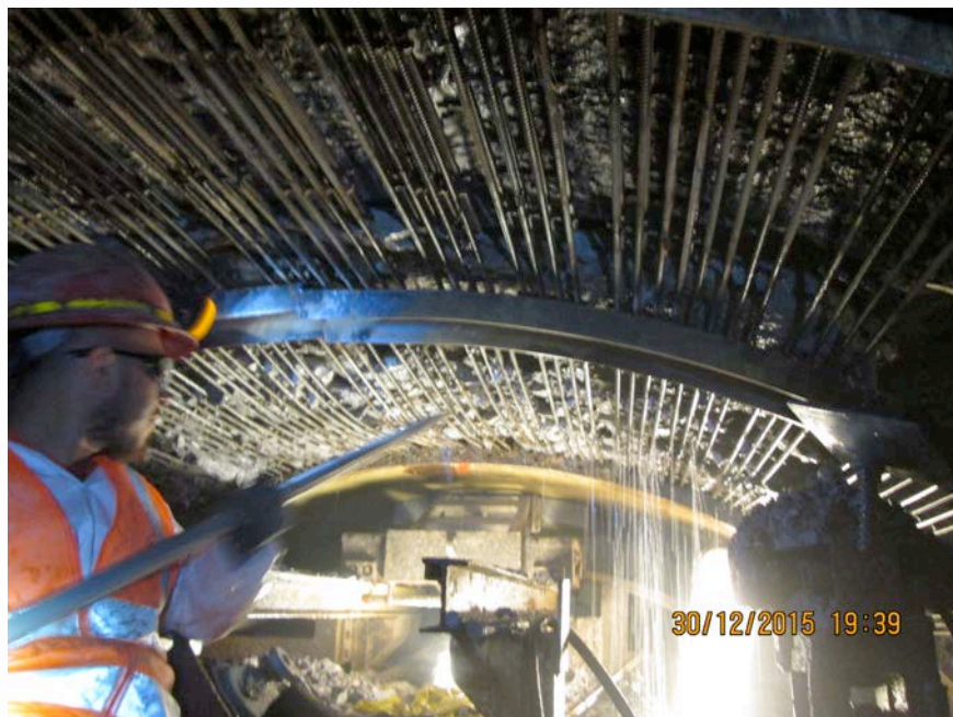
Fig. 14: Heavily sheared rock with high water ingress supported by flexing McNally system in the V5 EL Volcan tunnel (Ch 13.248).
