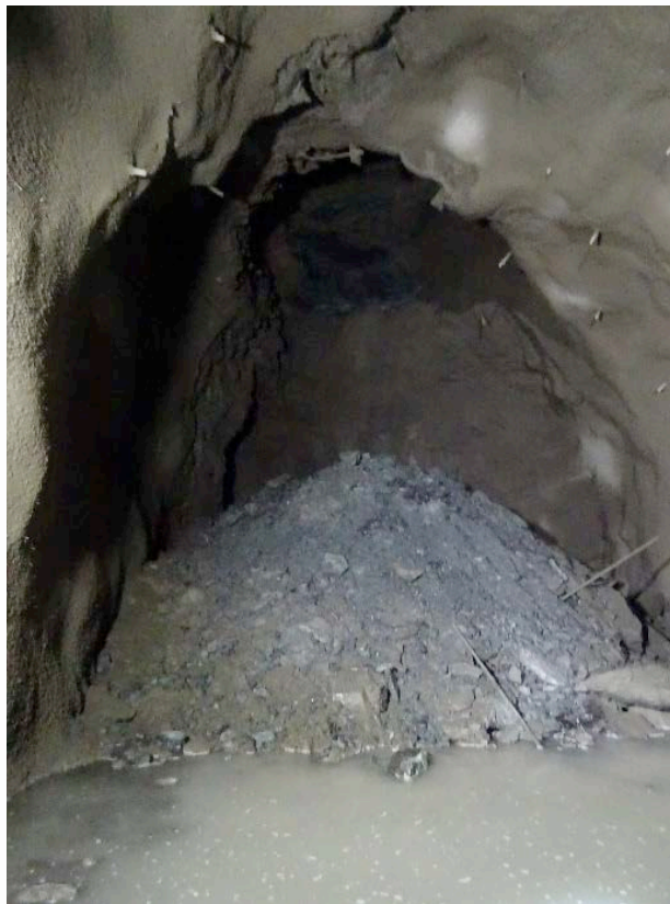
Fig. 18: Sudden collapse in the Alfalfal II tunnel (VA4) at Ch 0+553.
