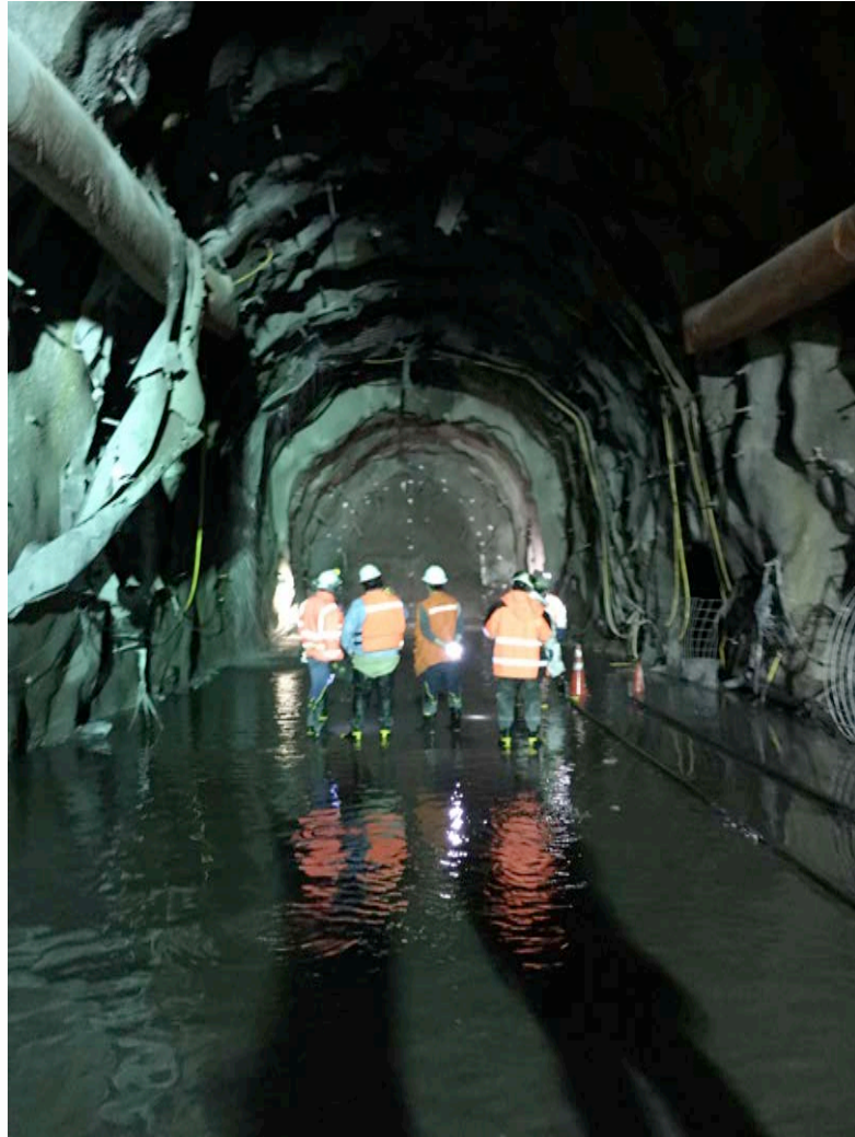
Fig. 17: Visit of El Volcan Tunnel V5 on 2. April 2017 observing water inflow rates of approx. 10-15l/sec.
