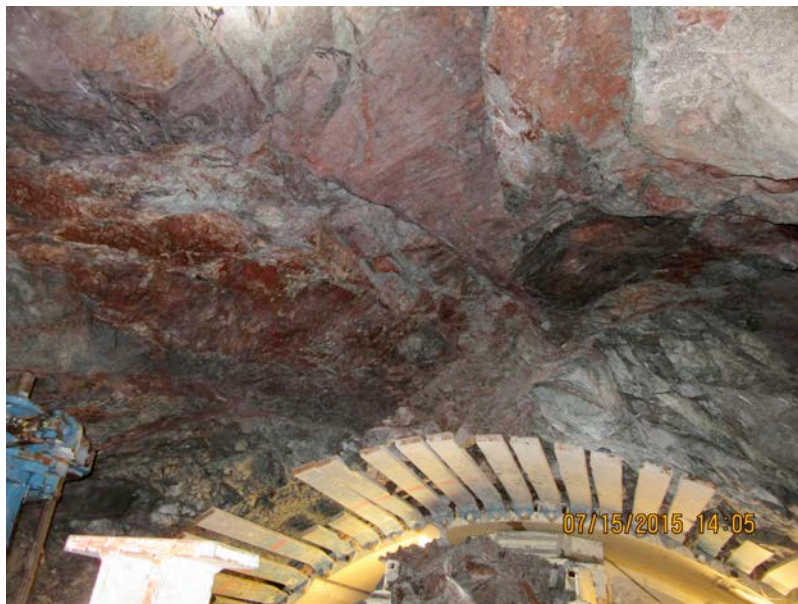
Fig. 9: Huge overbreaks above finger-shield in the V5 EL Volcan tunnel (CH 13.883).
