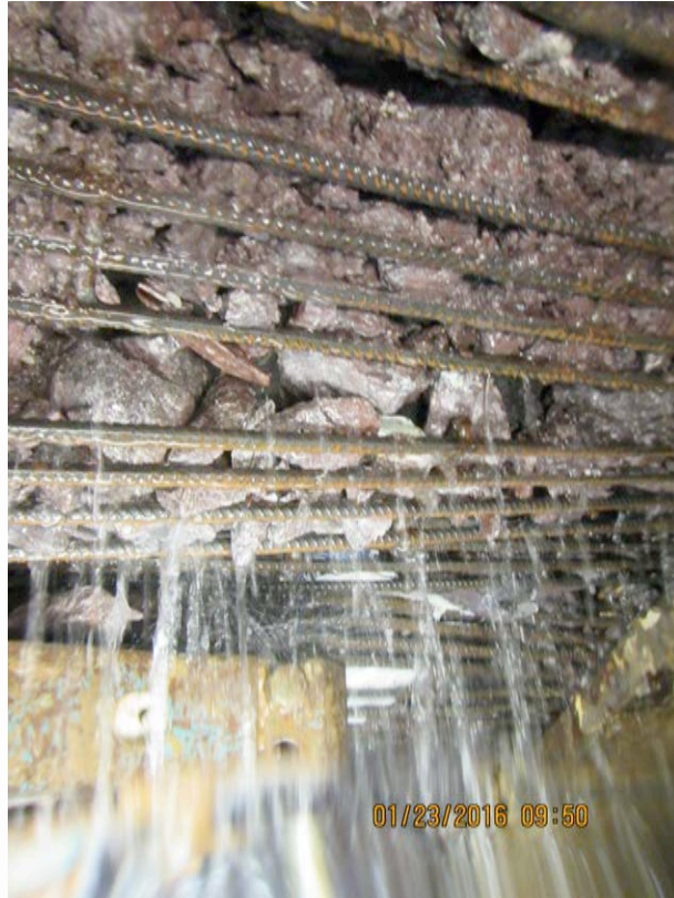
Fig. 14: Heavily sheared rock with high water ingress supported by flexing McNally system in the V5 EL Volcan tunnel (Ch 13.248).
