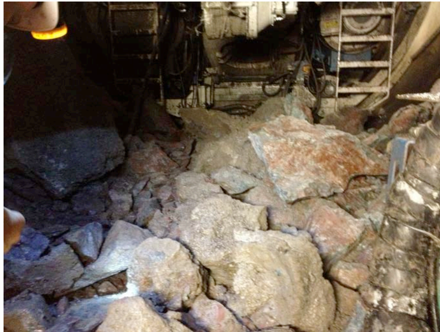
Fig. 12: Massive rockfall debris from overbreaks within L1-area in the V5 EL Volcan tunnel (CH 13.884).
