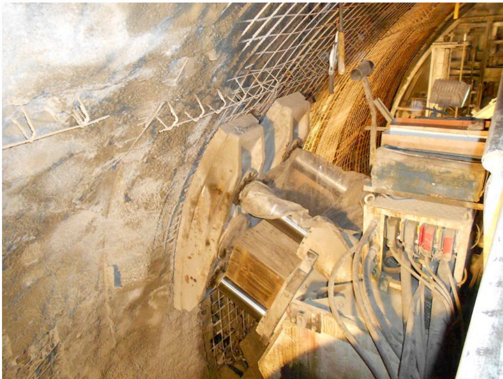
Fig. 6: Example of an open gripper-TBM in Switzerland with improved rock conditions under gripper-pads to provide stable abutment.
