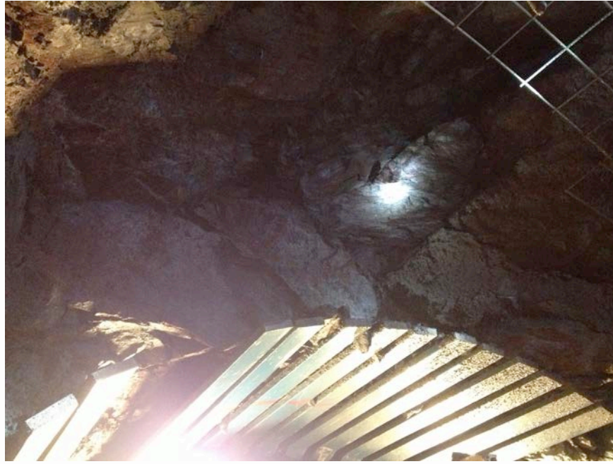
Fig. 10: Huge overbreaks above finger-shield in the V5 EL Volcan tunnel (CH 13.884).
