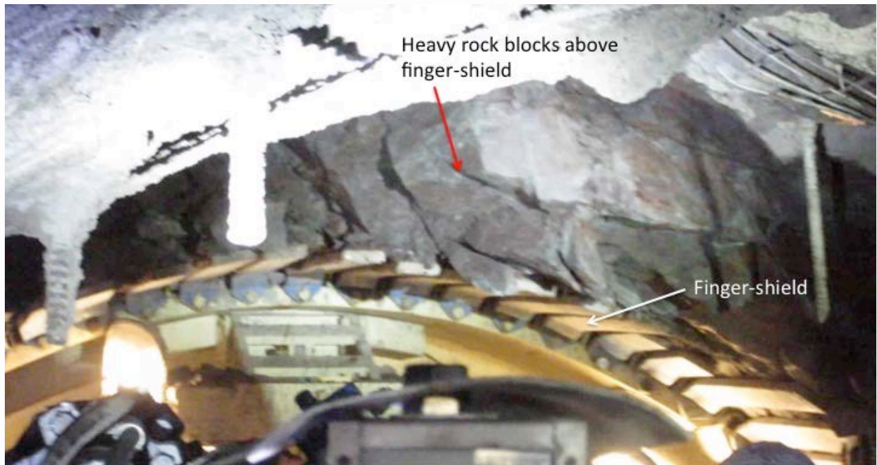
Fig. 3: Situation on gripper-TBM in El Volcan tunnel V5 at CH 13+883 with fractured rock blocks above finger-shield.
