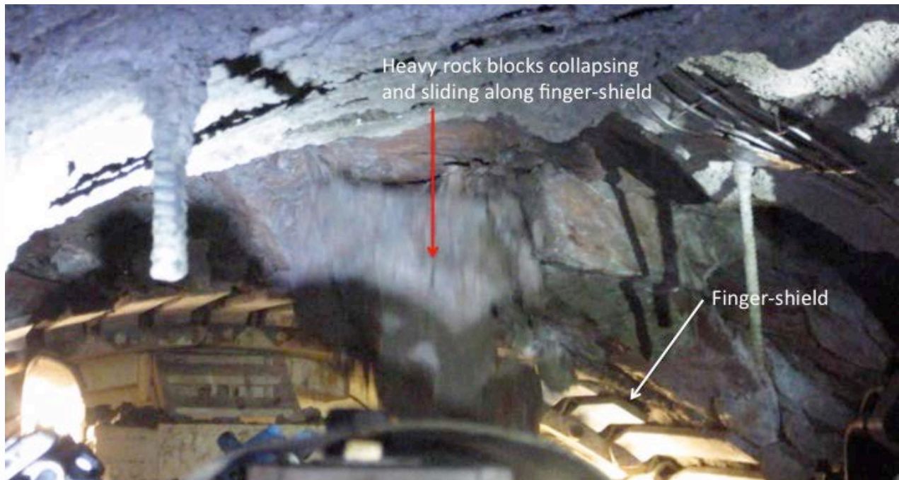
Fig. 5: Situation on gripper-TBM in El Volcan tunnel V5 at CH 13+883 with fractured rock block s collapsing and sliding along finger-shield.
