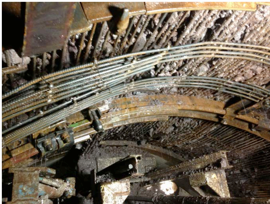
Fig. 13: Heavily sheared rock supported by the McNally system (which flex under the heavy load) in the V5 EL Volcan tunnel (Ch 13.250).
