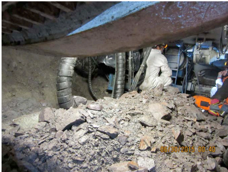
Fig. 11: Massive rockfall debris from overbreaks within L1-area in the V5 EL Volcan tunnel (CH 13.887).
